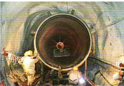
Installation of FRP pipes
